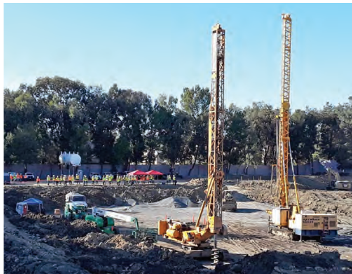
Field visit to observe vibro pier installation.
