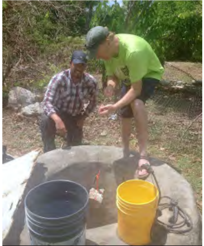
Installing a gauge in a well
