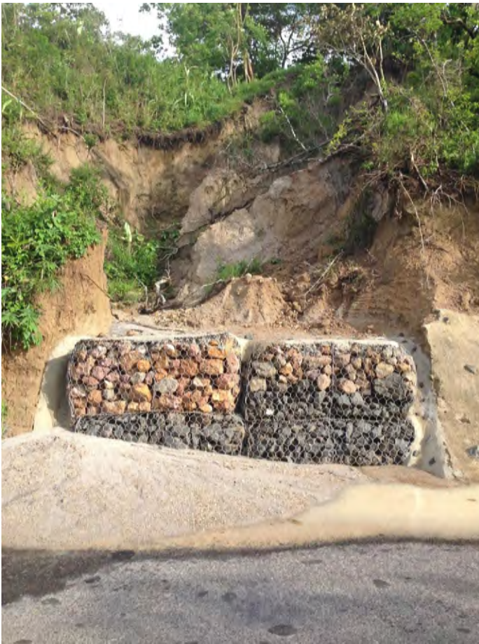
View of recently installed gabion wall below primary landslide
