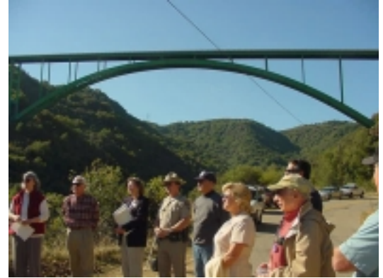
View of the bridge from the plaque site.
