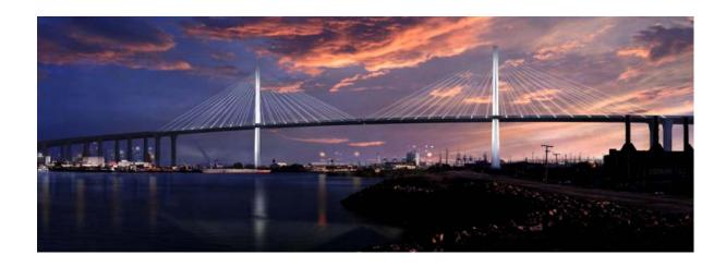
The Port of Long Beach is also impressive with the 44-year old Gerald Desmond Bridge about to be replaced with an iconic cable stayed bridge. Five hundred foot tall main towers will support a one thousand foot long main span.
