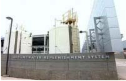
Orange County Wastewater Purification facility, Fountain Valley, Calif.
