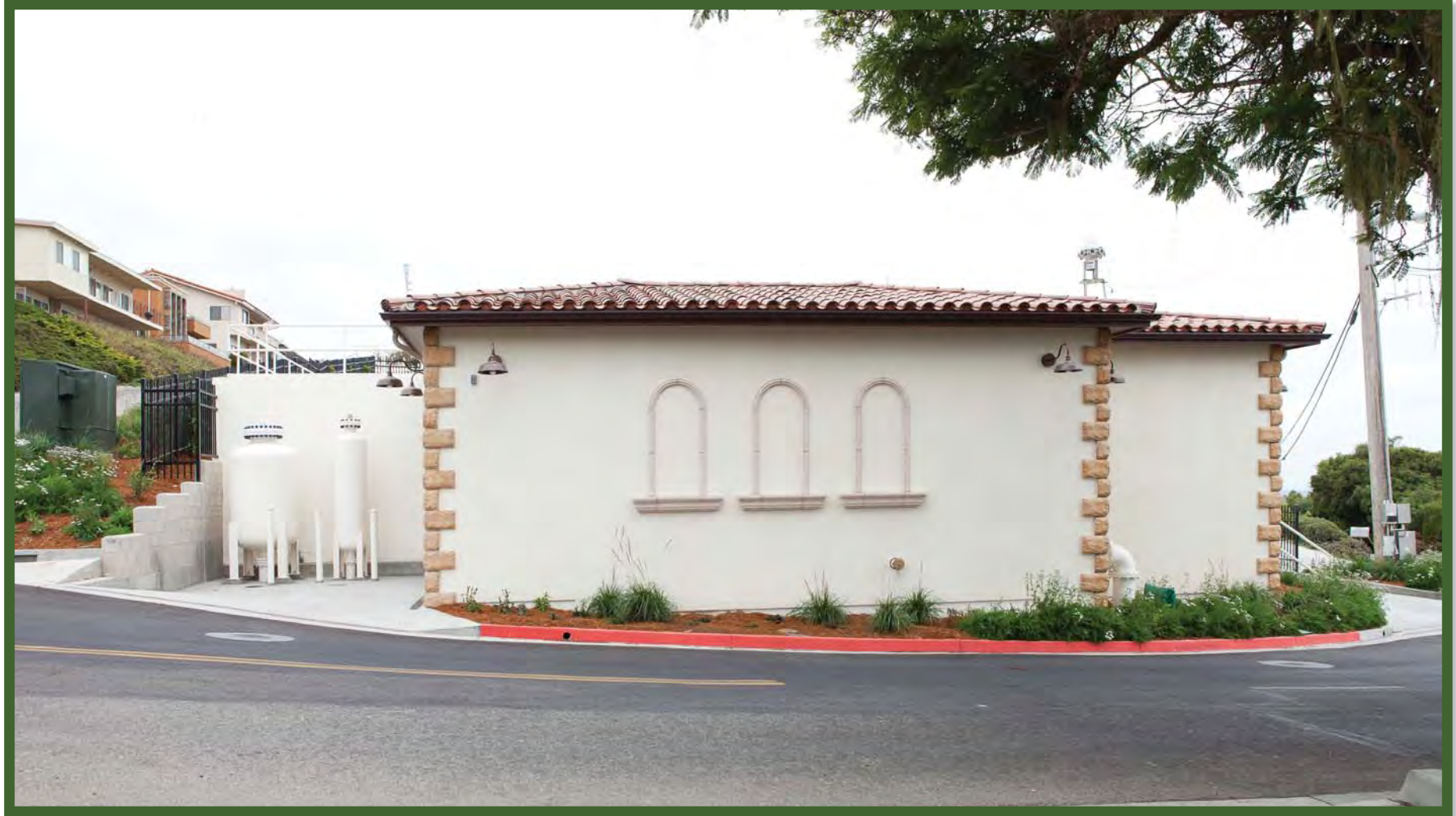
Pismo Heights-Finished Construction: Side view of the new booster station building with the second driveway and the two hydro-pneumatic tanks to assist with stabilizing system pressures and water hammer.
