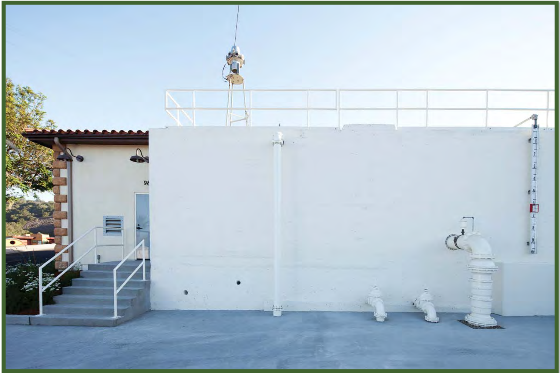
Pismo Heights-Finished Construction: Front face of the old tank and the access door to the booster station building.
