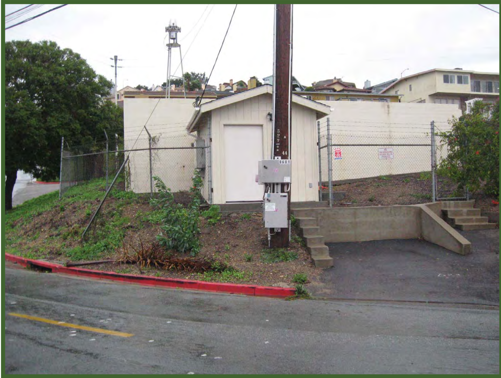
Pismo Heights-Before: Front of Tank and Booster Station, looking north. Operator's parking stall in front.
