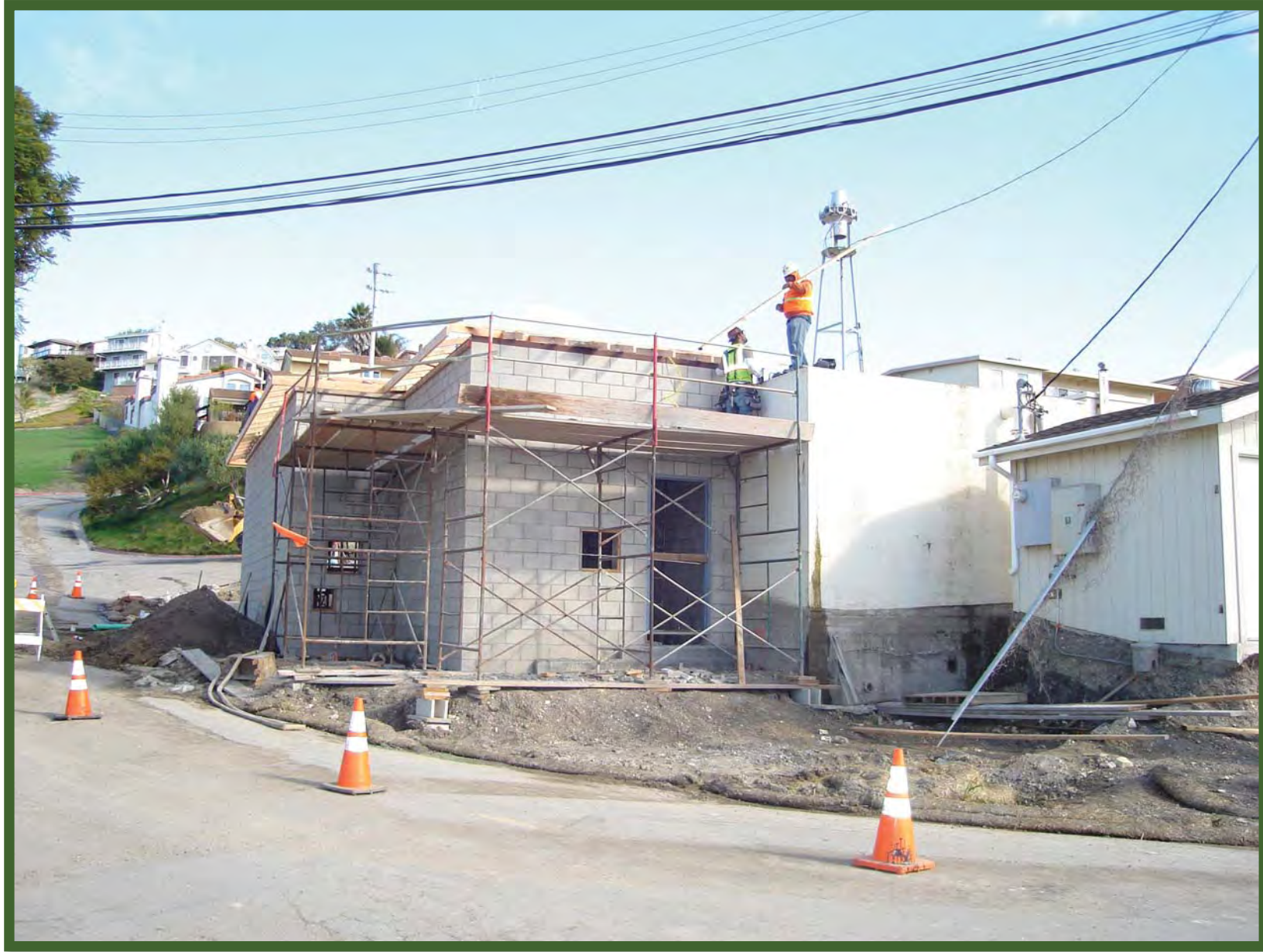
Pismo Heights-During Construction: Construction of the new booster station building. Note the existing booster station building still sitting on its foundation with the ground graded out around it.
