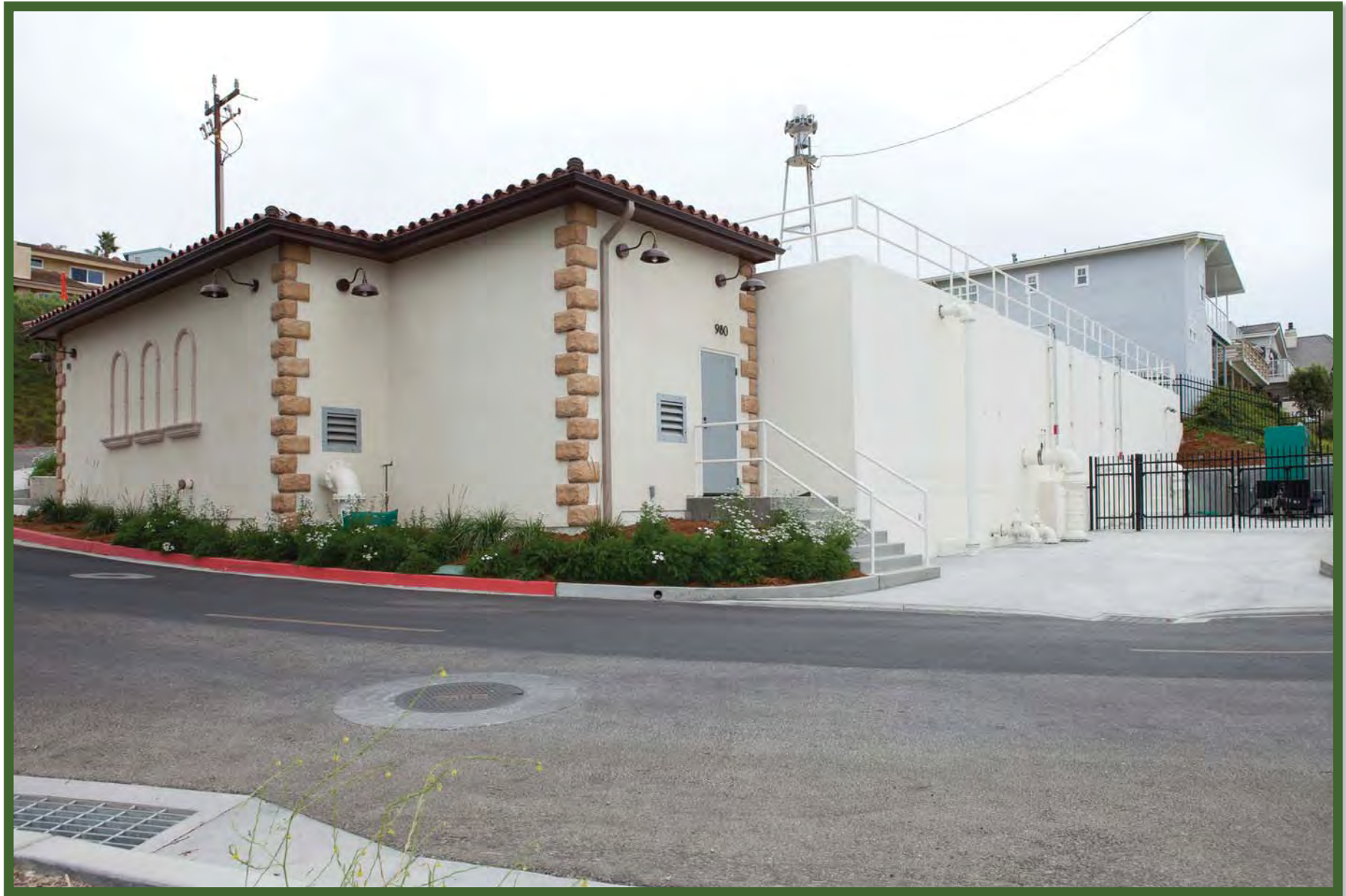
Pismo Heights-Finished construction: Front of the site was lowered 4 to 9 feet. Both tanks were painted and guard rail installed at the top of the tank. The generator is located at the back of the property behind the wrought iron fence.
