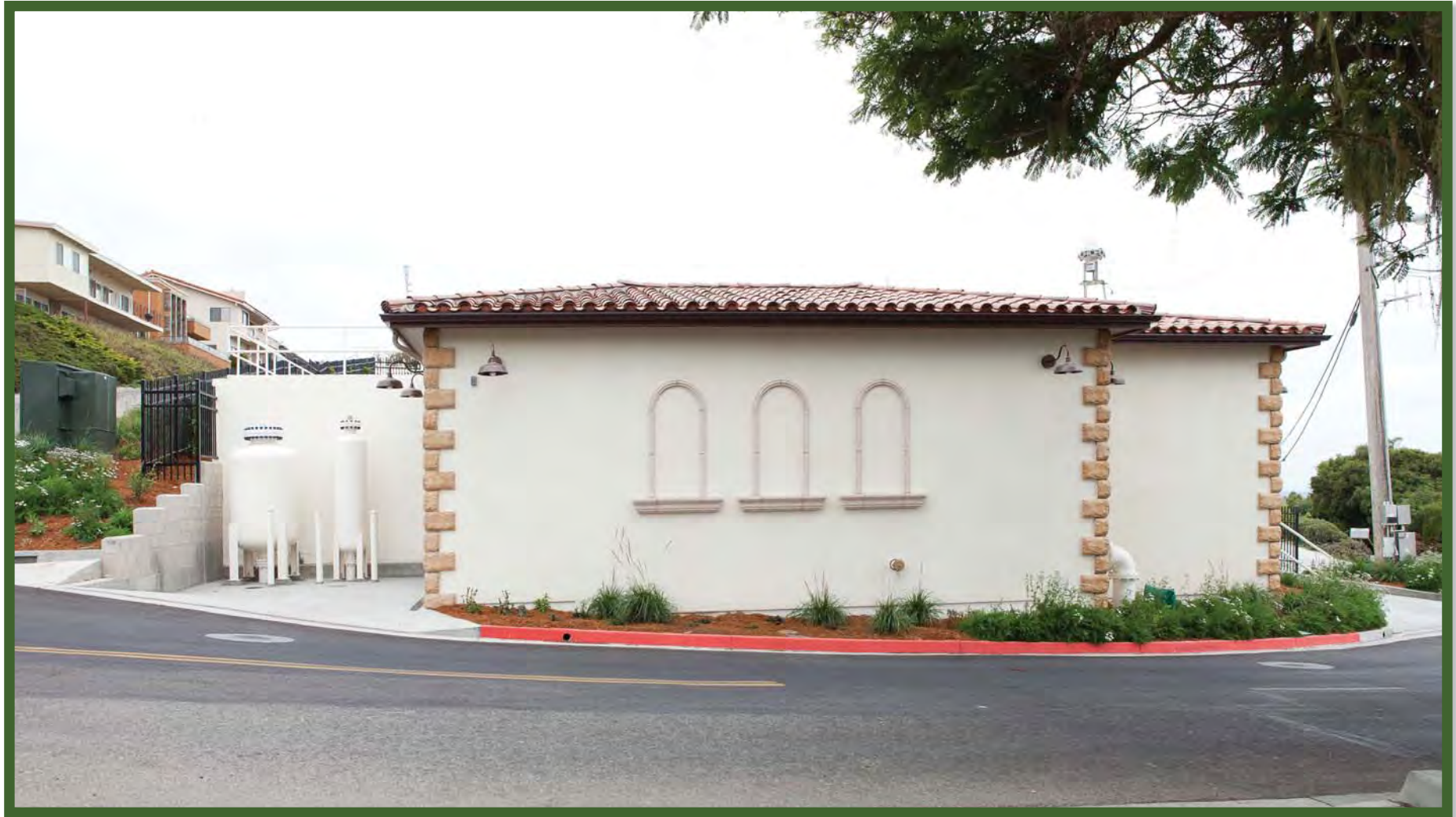
Pismo Heights-Finished Construction: Side view of the new booster station building with the second driveway and the two hydro-pneumatic tanks to assist with stabilizing system pressures and water hammer.
