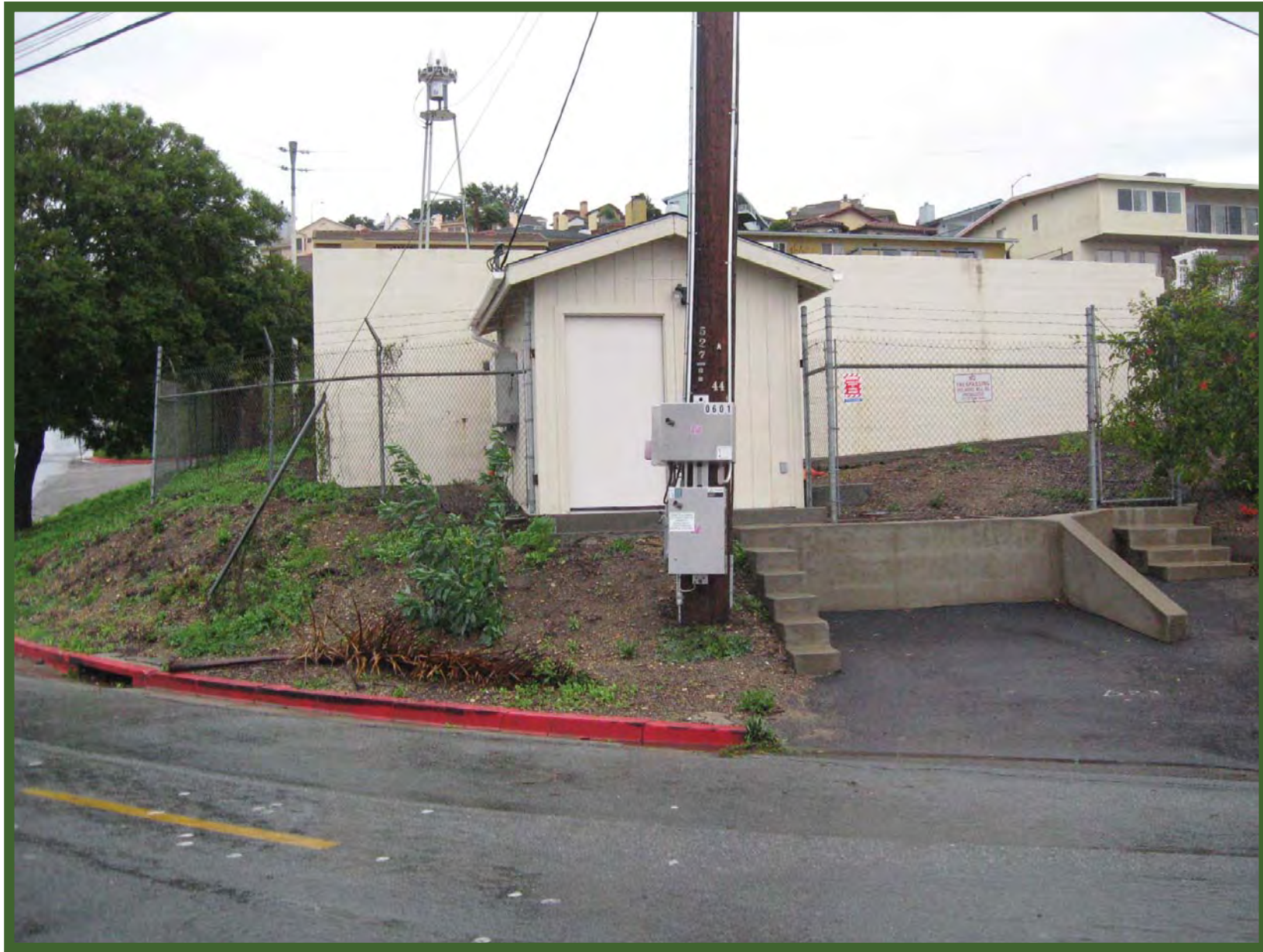
Pismo Heights-Before: Front of Tank and Booster Station, looking north. Operator's parking stall in front.
