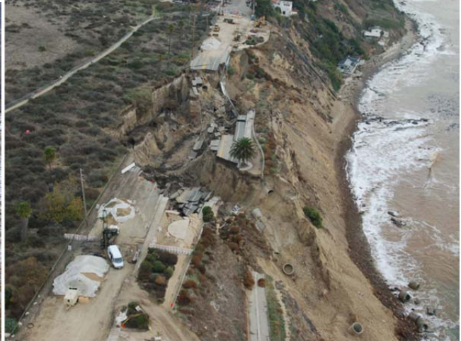
Post-Landslide (looking east along Paseo Del Mar)
