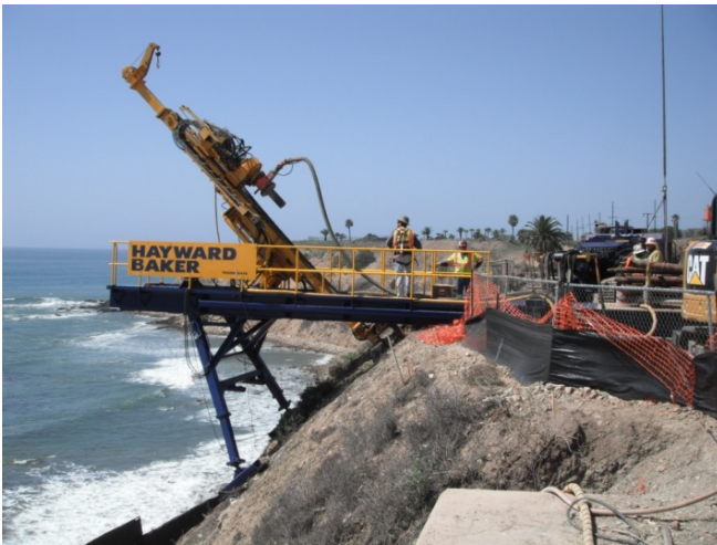
Anchor Drilling using Air Rotary Drill Rig
