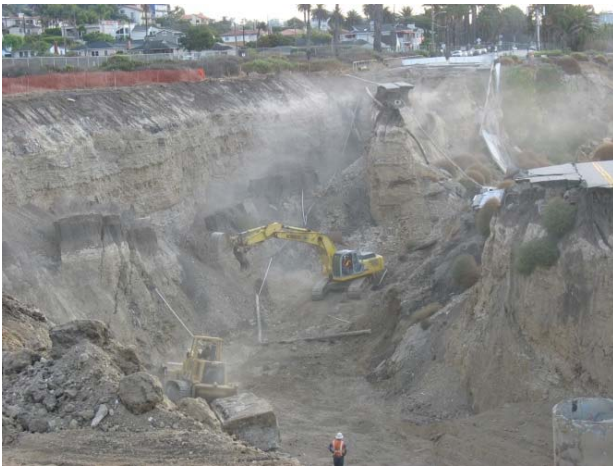
Demo / Grading (looking east)
