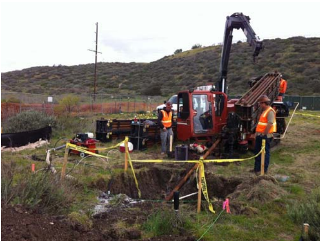
Horizontal Directional Drilling Entry Pit
