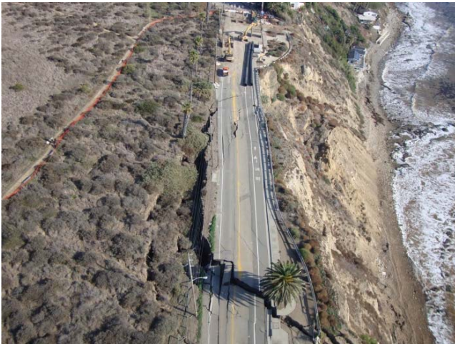
Pre-Landslide (looking east along Paseo Del Mar)
