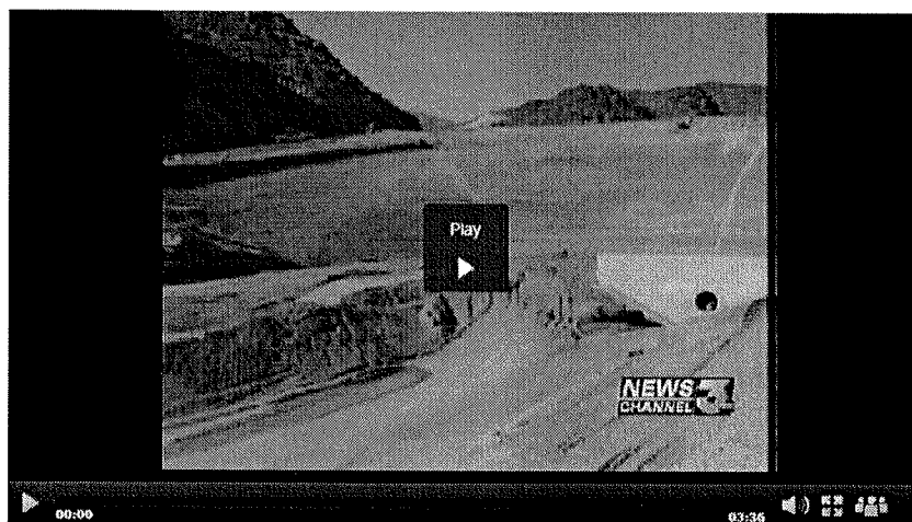
Eagle Canyon Dam nears completion
