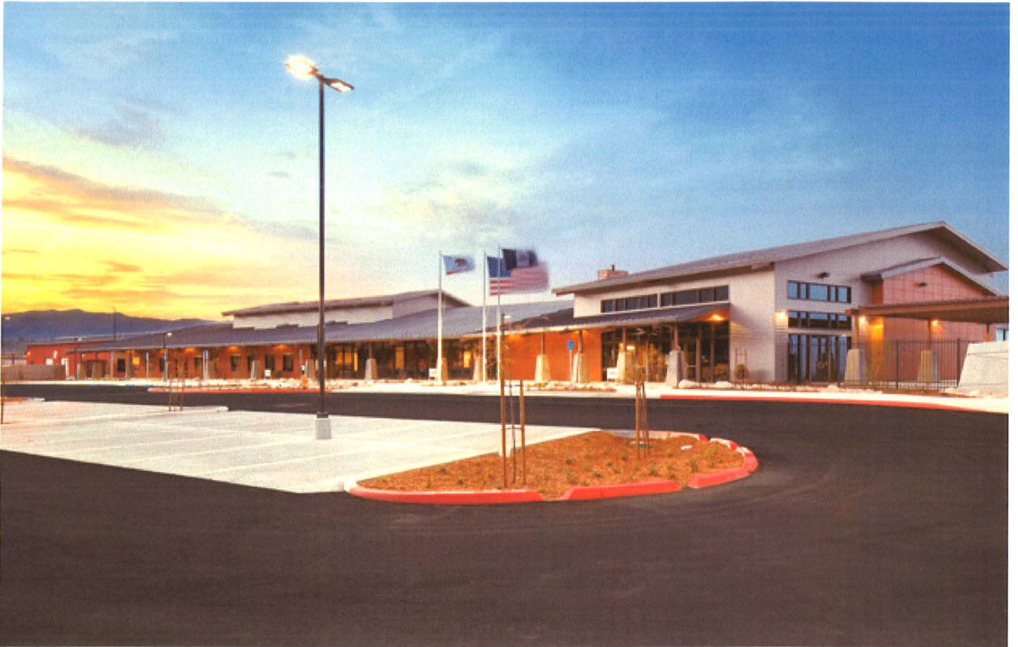
North Parking Area with Pervious Concrete Pavement
