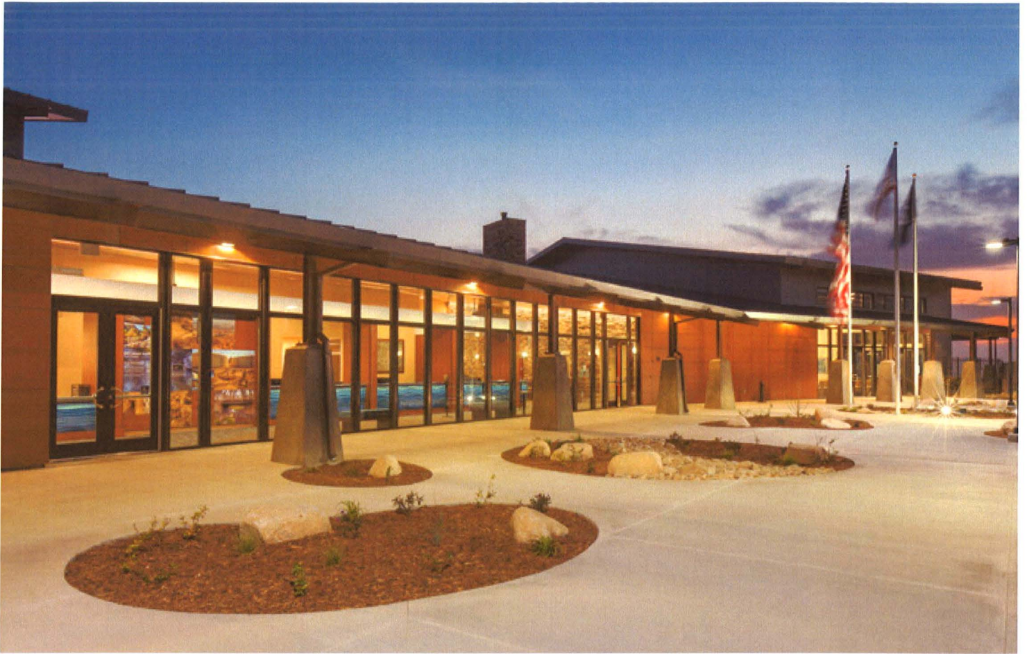
North Side of Administration Building - Main Entrance
