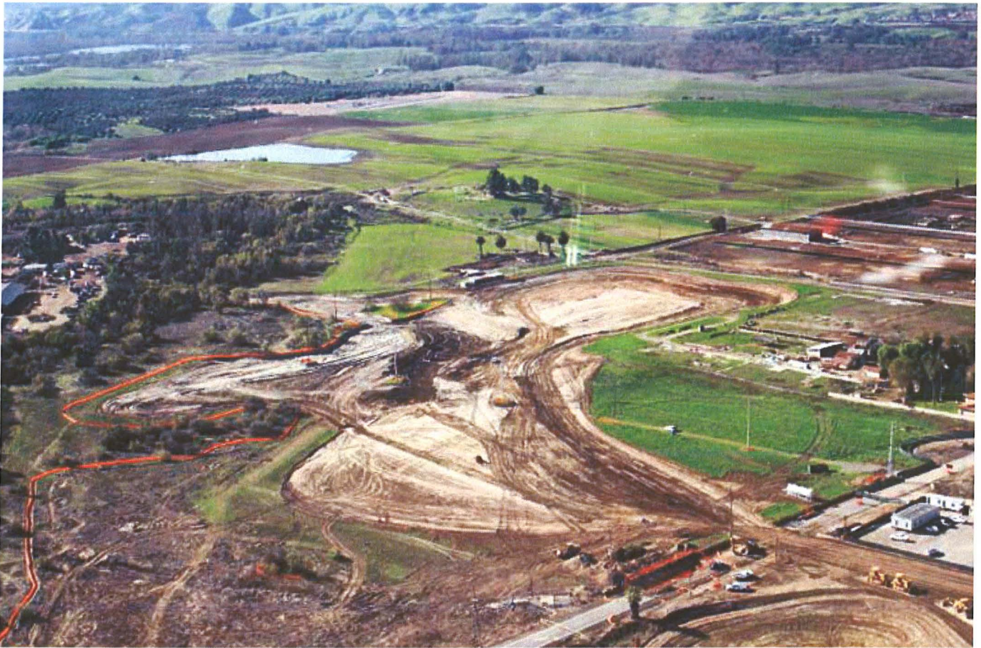
FIGURE 1. MILL CREEK WETLANDS PROJECT SITE BEFORE CONSTRUCTION.
