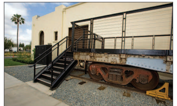
A dining area on the side of the building is constructed from two flatbed rail cars.
