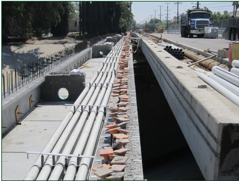
Utility Relocation Improvements on North Sidewalk (May 2012)
