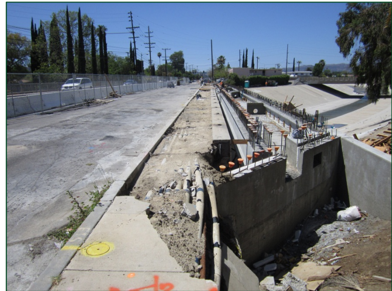
Demolition & Relocation of North Sidewalk (April 2012)
