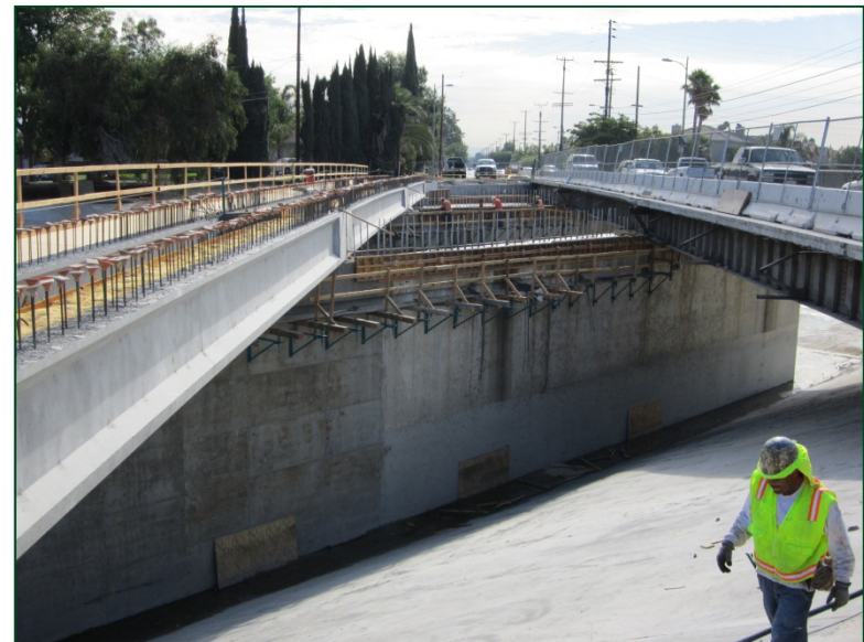
Demolition of Existing Bridge Deck (August 2012)
