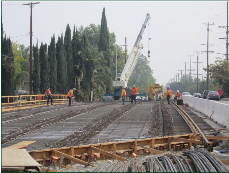
Construction of Reinforced Concrete Bridge Deck (November 2012)
