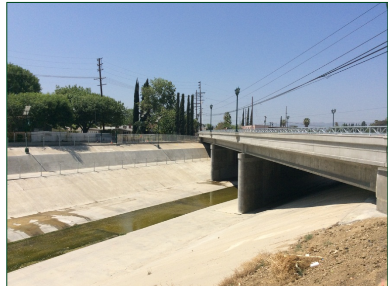
Newly Completed Vanowen Bridge Over LA River (April 2014)
