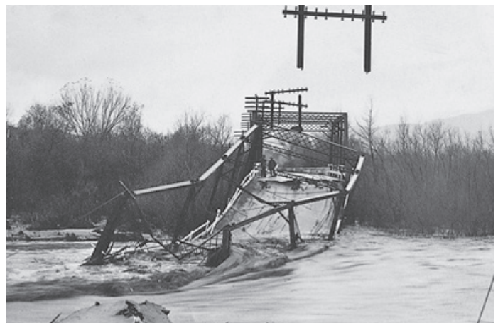
Bridge collapse on the Santa Ana River in 1916
