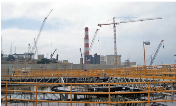
Secondary settling tanks at Hyperion Wastewater Treatment. Power plant in the distance currently supplies the Hyperion Plant. In the future Hyperion will supply all its power produced from treated digester gas
