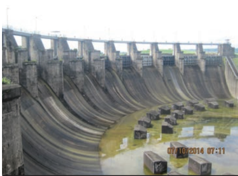
Gatun Dam Original spillway with 14 gates within the 1.4 mile long x 0.4 mile wide (at base) x 85 foot high
