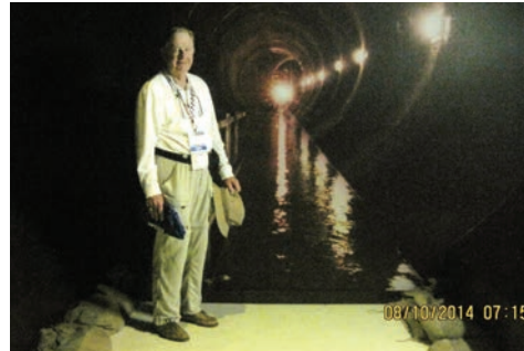
A typical massive, lock interior, culvert that controls inflow/outflow of water by gravity to raise and lower the ships. Currently 53 million gallons are used per ship passage. New locks will reuse two fifths less water.
