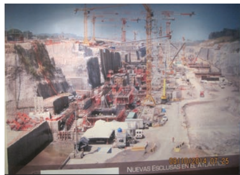
Rock excavation for Third Lane Lock on Atlantic side. Soft excavation is available on the Pacific side.
